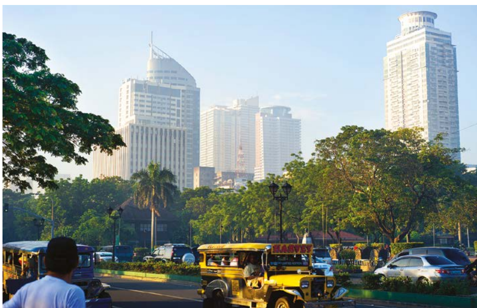
In the first half of 2014, commercial constructions accounted for about 45% of total flat glass demand.
