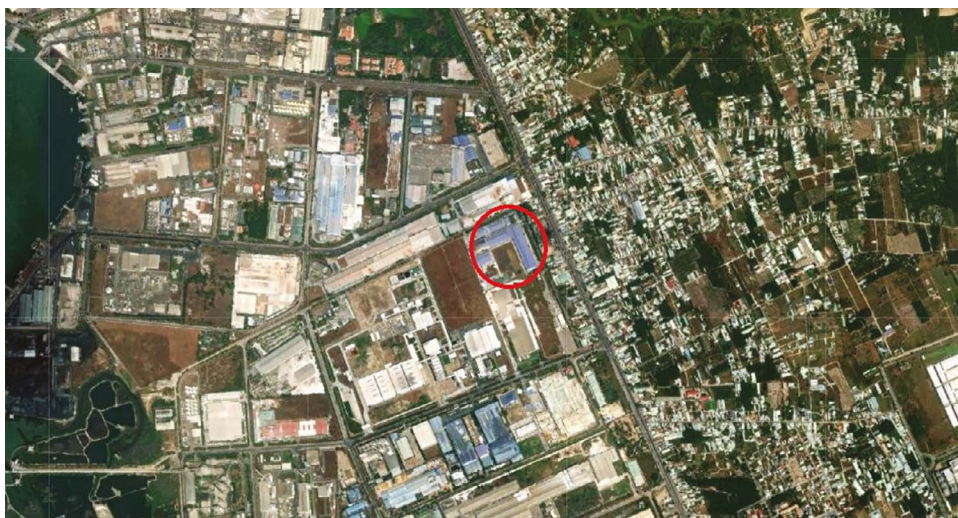
Aerial view of O-I BJC Vietnam Glass (circled in red) located southeast of Ho Chi Minh City in the My Xuan A Industrial Zone. The facility produces “nearly 300 million glass bottles [p.a.] for beverage, beer, wine, food and pharmaceutical products”, according to a company statement. Photo provided courtesy of the United States Geological Survey, 2022.
