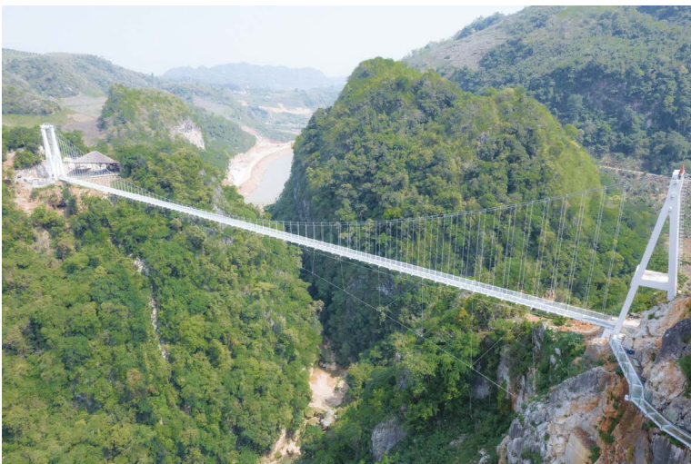
The Bach Long Bridge is located in the Moc Chau District of Son La Province in Vietnam. Photo provided courtesy of Moc Chau Island Mountain Park and Resort, 2022.
